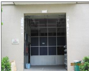
External photo(s) of the production unit(s) Factory gate on the 1st floor.JPG
