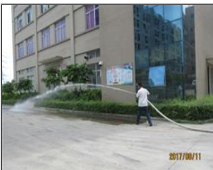
External photo(s) of the production unit(s) Fire hydrant testing.JPG
