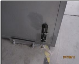
External photo(s) of the production unit(s) NC 7.15 Remark Locking device installed at the sliding door to keep opening durign working time 2.JPG
