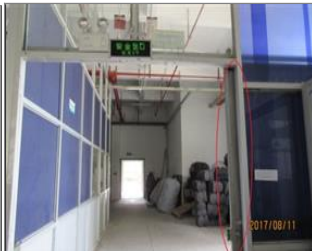
External photo(s) of the production unit(s) NC 7.15 Sliding door used at the safety exit in the cutting workshop 1.JPG
