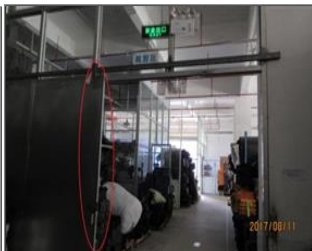
External photo(s) of the production unit(s) NC 7.15 Sliding door used at the safety exit in the cutting workshop 2.JPG
