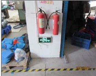
External photo(s) of the production unit(s) Evacuation sign in the workshop.JPG
